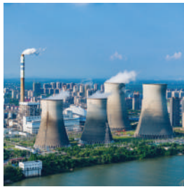
Thermal Power Plants
